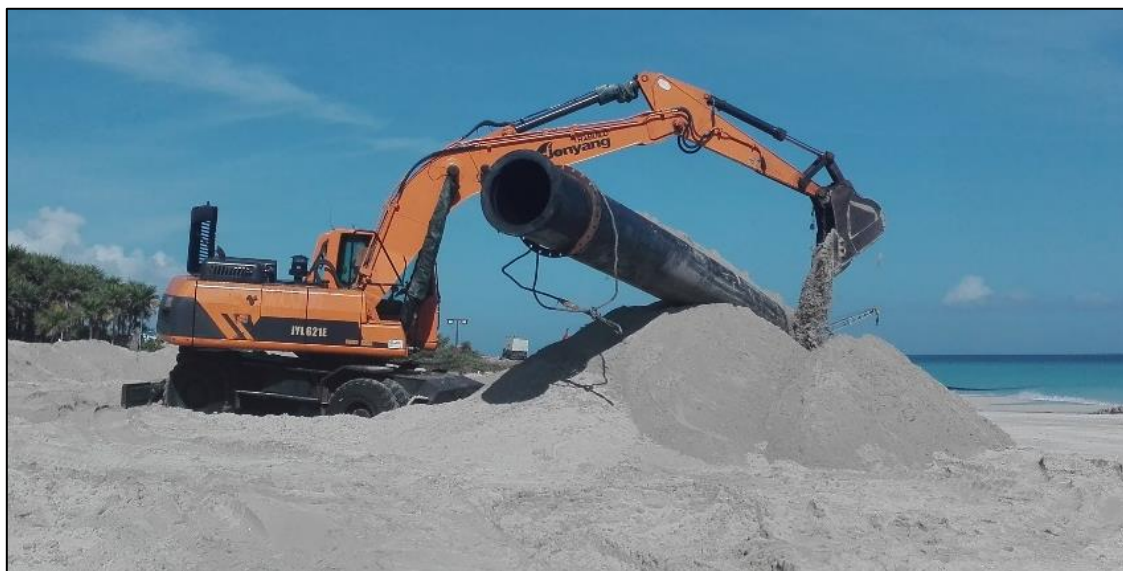
Photo 19: Backhoe placing pipe end at discharge point.
