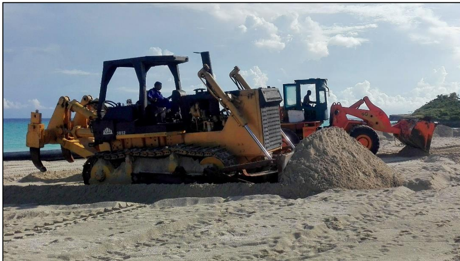
Photo 21: Leveling and conformation of the beach profile by mechanical equipment.
