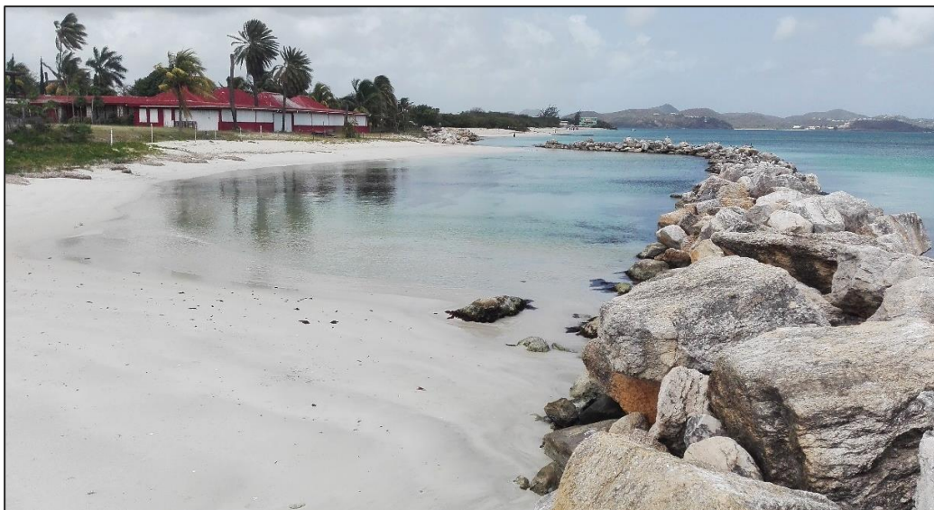
Photo 12: Behind the coastal defense structures in the central sector of Runaway Bay Beach, the low water circulation has caused eutrophication, proliferation of seagrasses and seabed stiffening.
